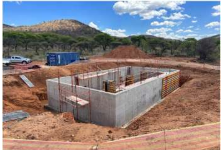
Pump Station 1 Concrete to Walls & Columns
